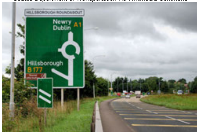
Transverse rumble strips alert drivers they are approaching a roundabout (Hillsborough, Northern Ireland)
