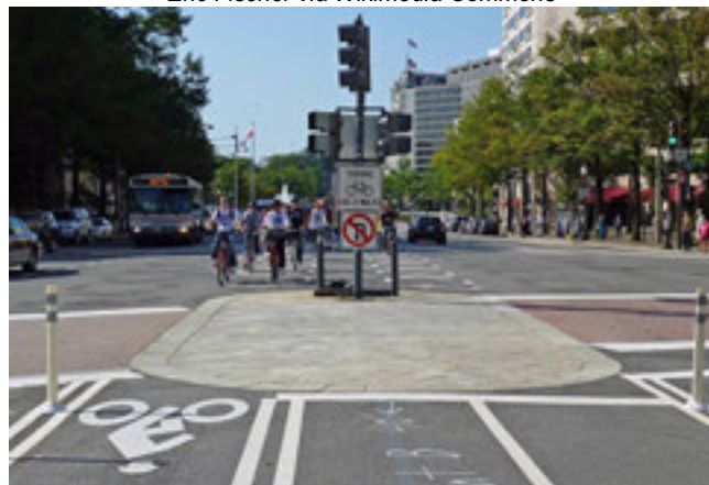
Left turns and u-turns are prohibited to allow cyclists and pedestrians to safely traverse the intersection (Pennsylvania Ave, Washington, DC) Payton Chung via Wikimedia Commons
