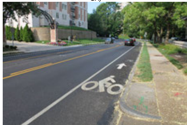
A four-lane road reconfigured to a two-lane road with a continuous turn lane and bike lanes (Lower Merion, PA) Montgomery Counting Planning Commission via Wikimedia Commons
