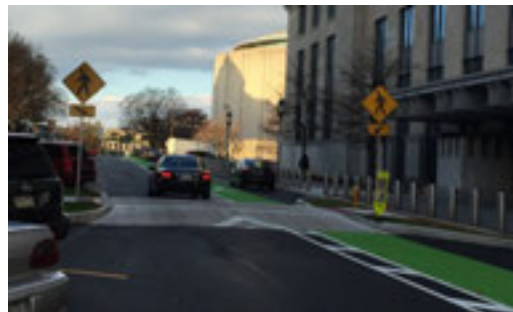
A raised pedestrian crossing with a sinusoidal slope, which reduces discomfort to cyclists and drivers (Harrisburg, PA) Pennsylvania Department of Transportation via the Pedestrian and Bicycle Information Center
