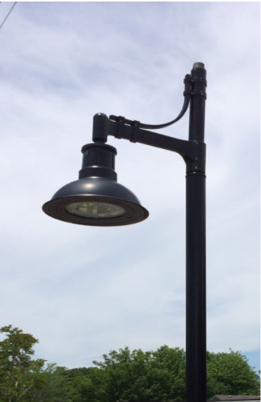
Pedestrian light components: Luminaire and pole - image represents general style, but not the exact fixture.
