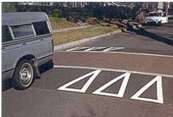
Asphalt speed table with stamped asphalt top and appropriate warning markings
